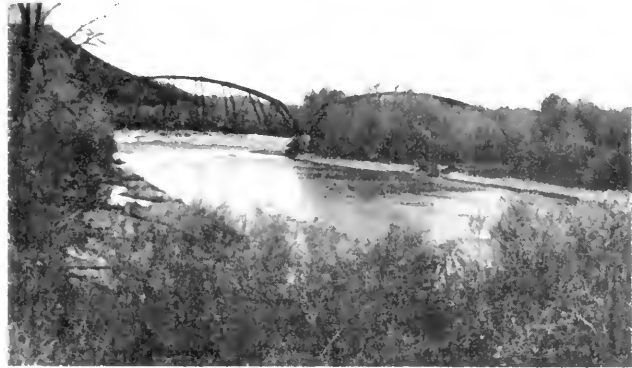
Present day railroad bridge over the South Fork can be seen east of the Twin Bridges. (Built in 1915.)
