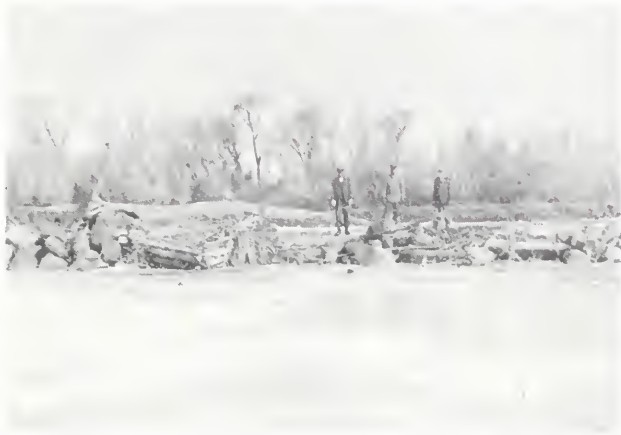
Riprapping on north bank of Snake River (South Fork). (Men unknown)
