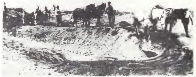
Working with Slip Scrapers on the John Taylor farm.
