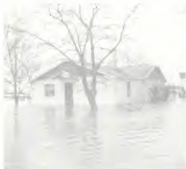
1962 flood Ross and Mary Buckland's home
