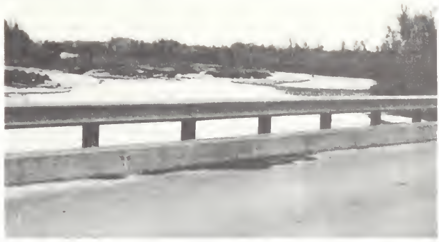
The second of the Twin Bridges.
